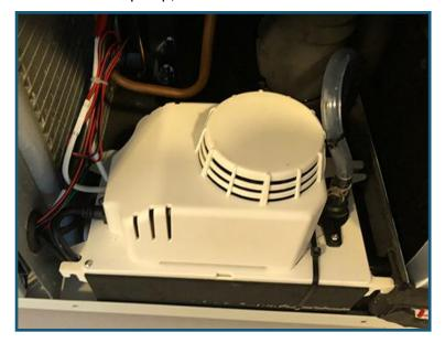
10. Pour clean water into the drain tray until you hear the pump energize twice (typically 16-32
