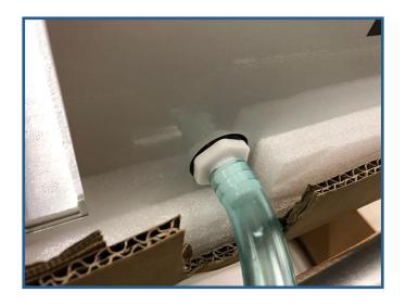
6. Slowly pour the cleaning solution into the drain tray, moving from side to side to evenly distribute it. *NOTE: If you get any of the cleaning solution on the coils, flush with water.*
