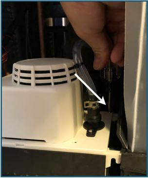
5. Use a flathead screwdriver to lift the pump head off the reservoir.
