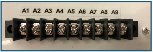
9. For fan interlock to function, place a jumper between A3 and A2. Next, connect terminal A1 on the dehumidifier to the remote fan terminal on the HVAC controller (normally terminal "G"). (see wiring diagram on next page)
